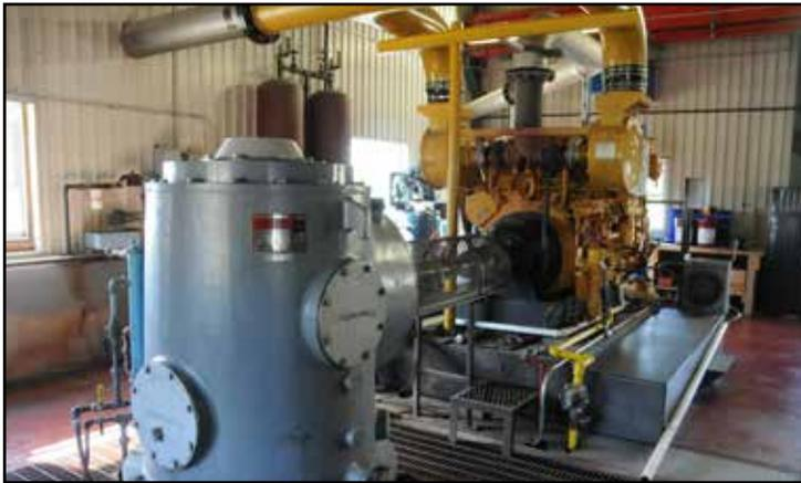
**60" pump with 825hp Diesel engine
