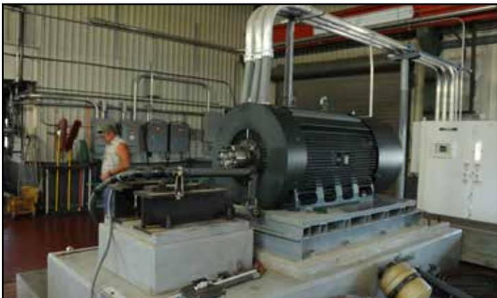
**42" pump with 600hp Electric motor
