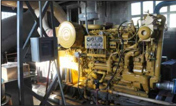
**60" pump with 905hp Diesel engine
