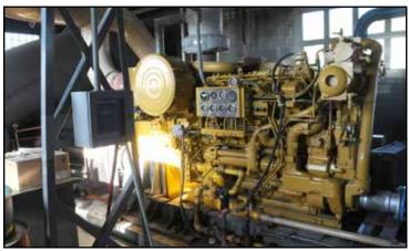
60" pump with 905hp Diesel engine pumping 115,000 gal/min.
