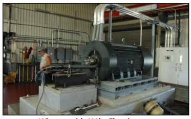
42" pump with 600hp Electric motor pumping 63,000 gal/min.
