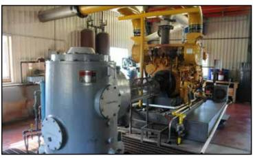
60" pump with 825hp Diesel engine pumping 97,000 gal/min.
