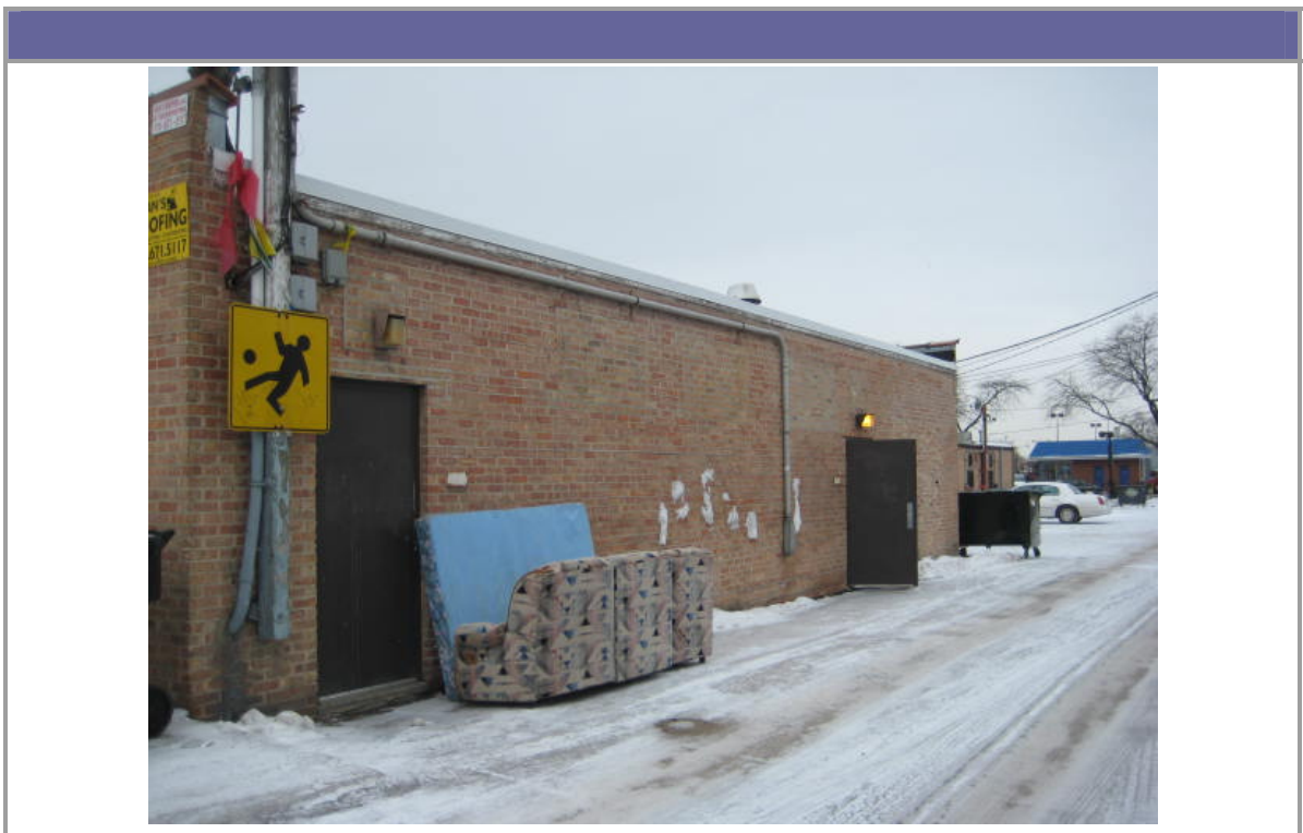
Exterior View of the Subject
