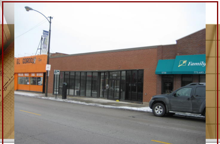
Photograph of Subject Property
