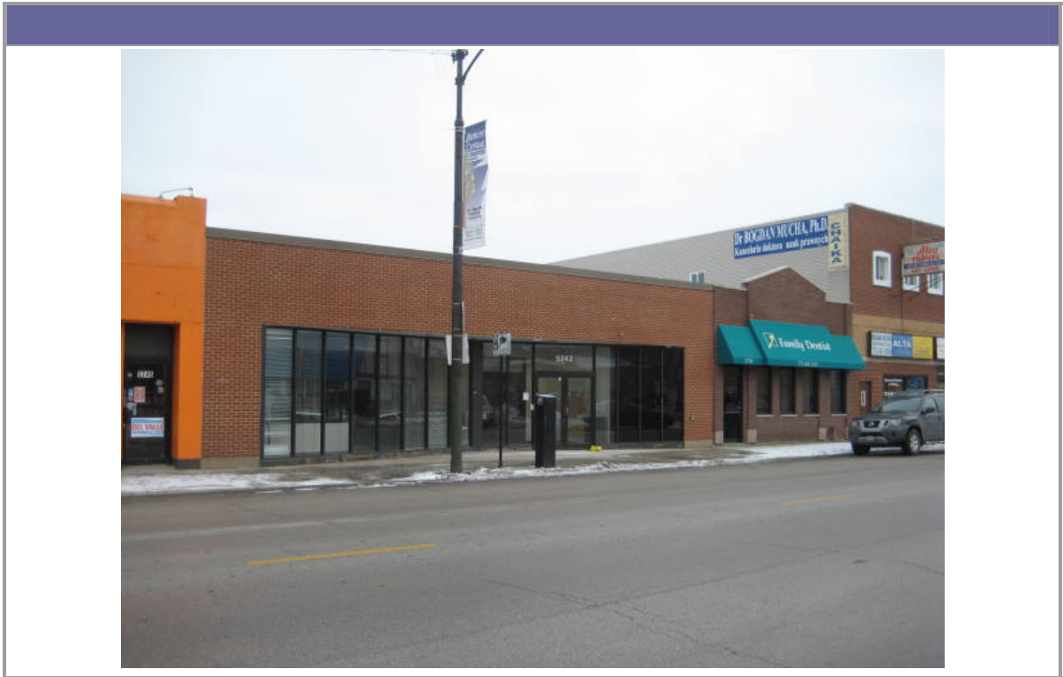
Exterior View of the Subject
