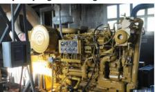
60" pump with 825hp Diesel engine pumping 97,000 gal/min.
