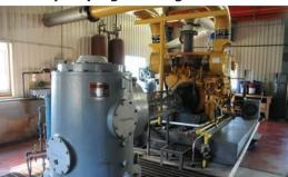
42" pump with 600hp Electric motor pumping 63,000 gal/min.
