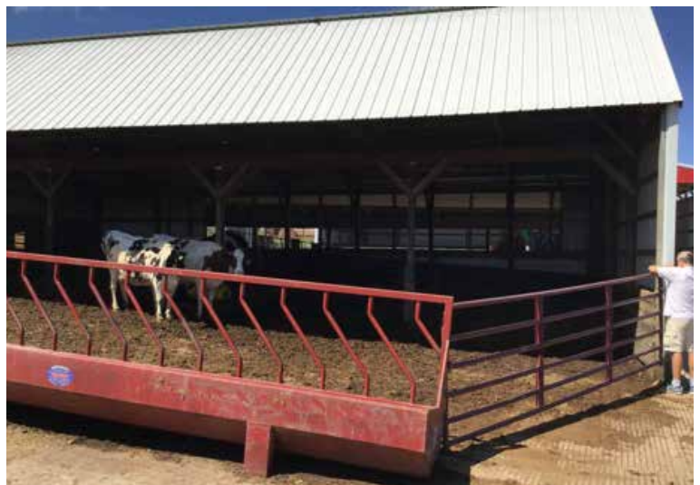
Dry Cow Barn - 42' x 56', Monoslope building 12' tall max height. Cement floor. 100 amp breakers. LED lighting. Ritchie frost free water. One cooling fan.
