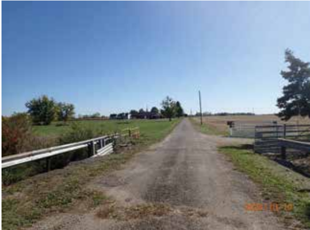
LOOKING SOUTH OF ROAD
