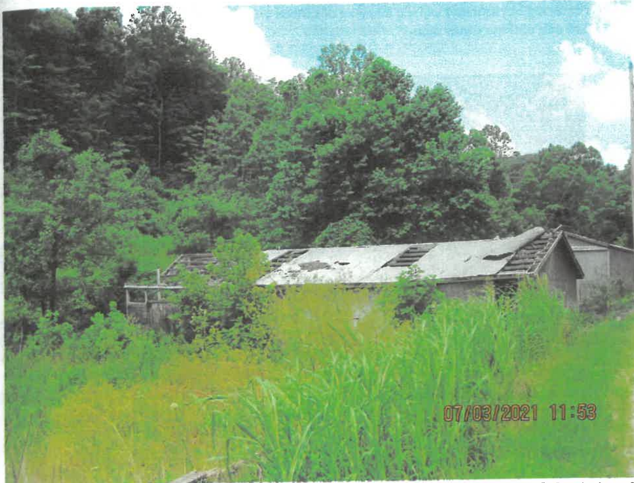
Structures along Carr's Run in Area C
