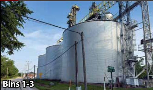
Bins 1-4 and Dryer System
