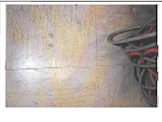
HA - 14/15: 12"x 12" Off white floor tile/mastic associated with 12"x12" off white floor tile
