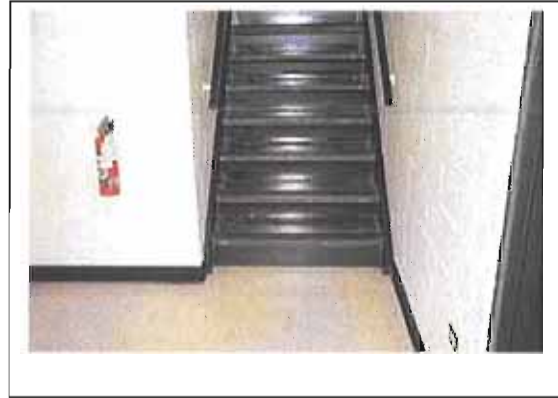
HA- 19/20: Stair treads in stairwell/mastic associated with stair treads
